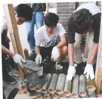
Students learning practical skills of construction by placing bamboo tubes layer by layer with mortar for the Dabao school and community centre project
